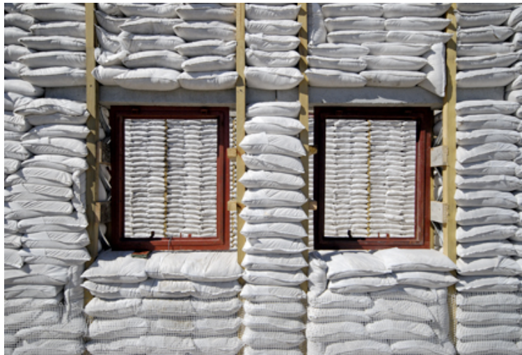
SANDBAGS HELP FORM THE STRUCTURAL CORE OF THE HOUSE.
